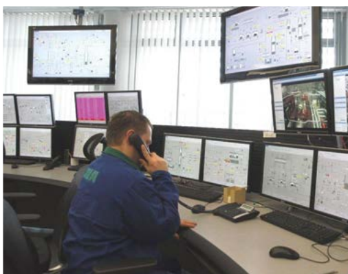
Figure 1: To produce fuels in compliance with EU environmental standards, INA Rijeka oil refinery in Croatia installed integrated control and safety systems in a centralized control room (above) on three units at its hydrocracking complex (top). Photo Credit: Emerson Process Management and INA Rijeka
