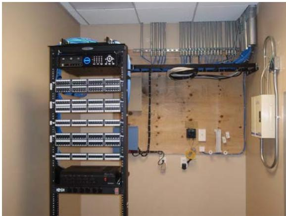
**5:** A Tier 5 Demarcation Point or Main Point of Presence where the external meets the internal interface.
