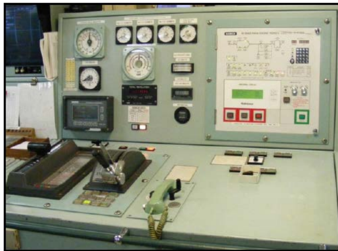
Figure 7: Vessel System and Engine Control Panels (on ship) 16
