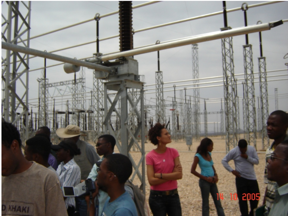
Fig. 3. A group of Polytechnic of Namibia students visit the AUAS 400 kV substation
